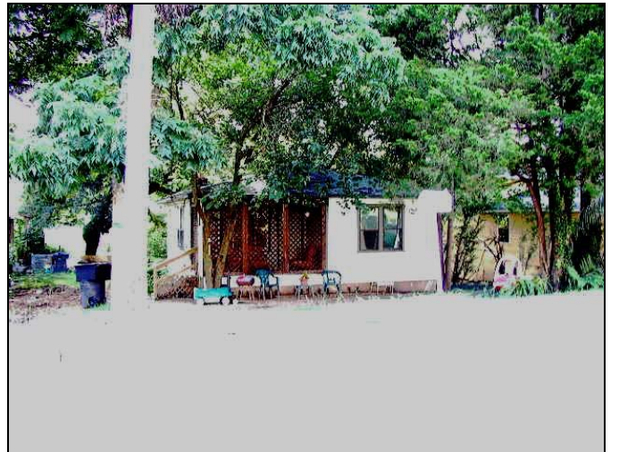
Case 5 After – 1213 Richmond – In August 2004, the front porch and the stairs had been repaired, toys were in the front yard and the house appeared to be in compliance.
