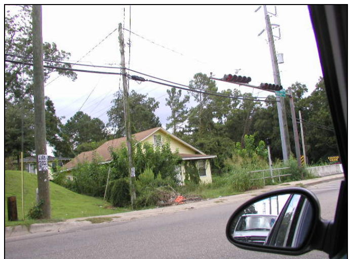
Case 7 – After – 1022 Railroad – In August 2004, the vehicle had been removed but the building was still overgrown with weeds, and the building was posted as condemned.
